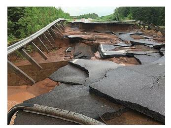
Figure 5. Damage along State Highway 23 near the South Fork of the Nemadji River in Carlton County, Minn., after flash flooding. Courtesy of Sgt. Jason Warnygora | Carlton County Sheriff's Office
