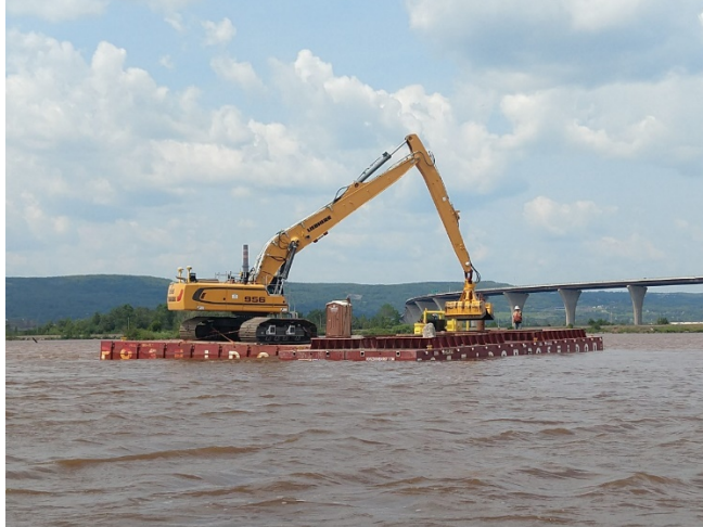
Figure 4. Sediment dredging and coastal marsh habitat restoration work at Kingsbury Bay was completed in 2021.
